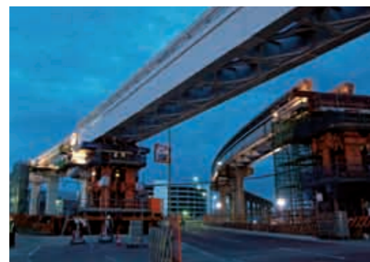
Relocation of monorail bridge
