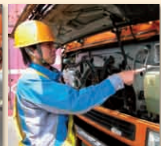
Air-conditioner gas status check using sight glass
