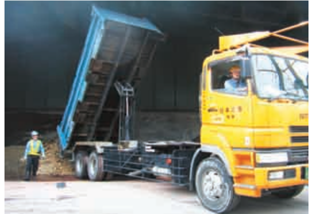
Sludge removal using open-top containers
